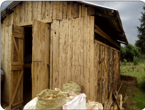
Diffused Light Store (DLS) made from local materials
