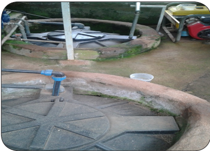
Aerponics unit construction system
